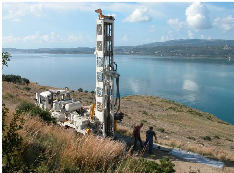
**Figure 1: Drilling the 122 metre (400 foot) test borehole**
